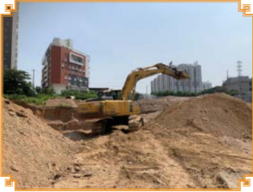
Basement Earth Work - Completed
